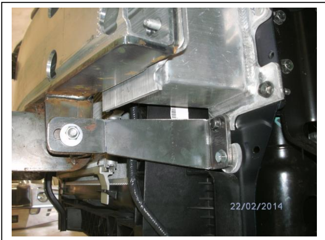
Figure 9: Lower mount support installed.
